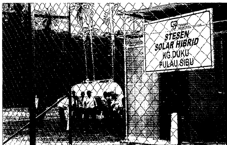
A Solar Hybrid Station at Pulau Sibul, Johor
