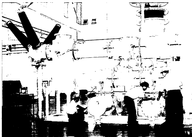
Maintenance and inspection works of GIS at TSG in progress
