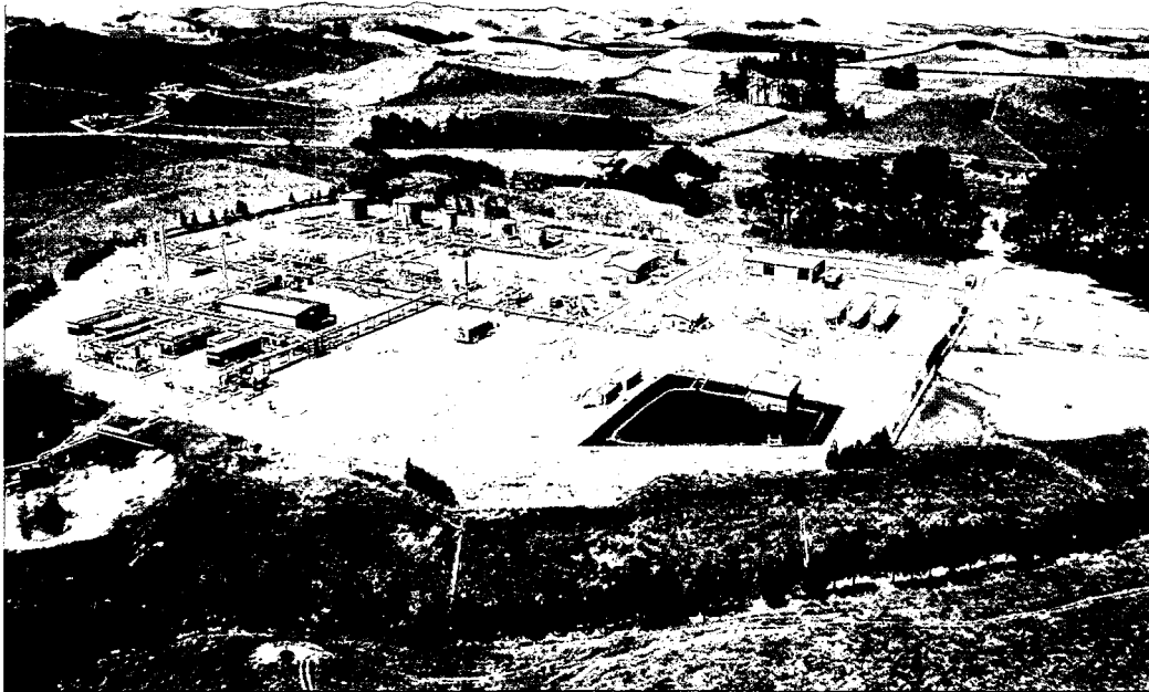
The TAWN Area's Waihapa Production Station consists of the Waihapa Oil Plant and the Tariki Ahuroa Gas Plant, with a combined capacity of 15,000 barrels of oil and condensate per day and approximately 40 MMcf of natural gas per day. In 2004, Swift Energy doubled the gas plant's capacity for extracting and processing liquid petroleum gases.
