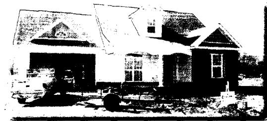
New Home Construction – Warner Robins
