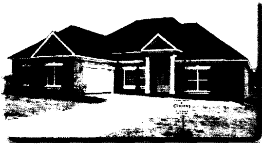
New Home Construction – Savannah
