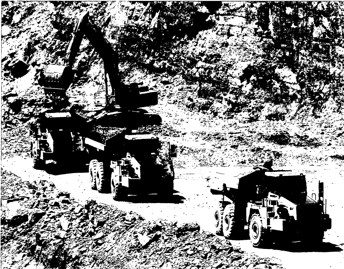
Workers at The Shelly Company's Marble Cliff Quarry in Hilliard, Ohio remove shot rock in preparation for expanding the mine to include an underground operation. A US$12 million capital expenditure project, the underground mine will allow Shelly to retrieve 90 million tonnes of high-quality friction-grade material while continuing its surface mine operation that produces non-friction commercial-grade material. The mine is scheduled to go underground in early-2006.
