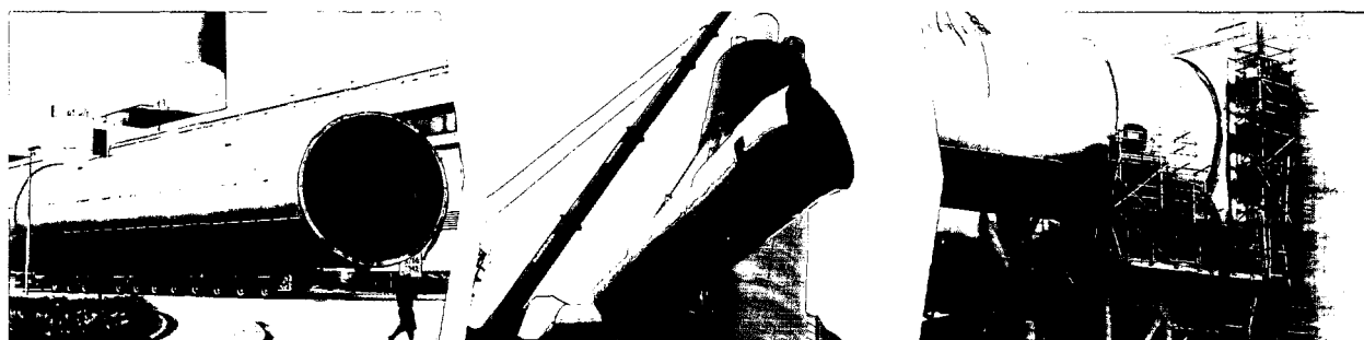
Transporting, fitting and testing an exhaust duct at Black Point power station
