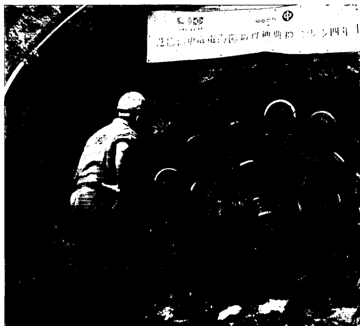
Breakthrough at the Chi Ma Wan tunnel on the south coast to the Long (CLP) cable project
