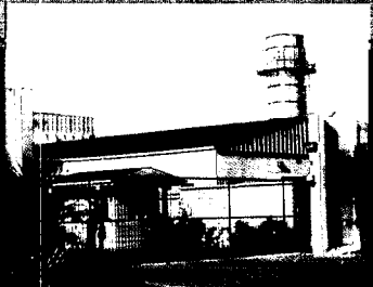
This electric generating facility is the newest and lowest cost electricity provider in Trinidad and Tobago.
