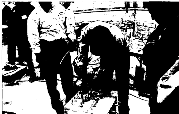
Concrete installers learn from Ray Magallanes, Brea Sales Representative, at a Spanish workshop on Adhesive Anchor Installation.
