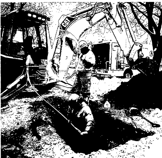
Utility crews work even in snowy and frozen conditions to improve the safety and reliability of the system by replacing old steel pipe with new plastic lines. This was the case here, at a residence in Tonawanda, N.Y., where gas service was renewed.
