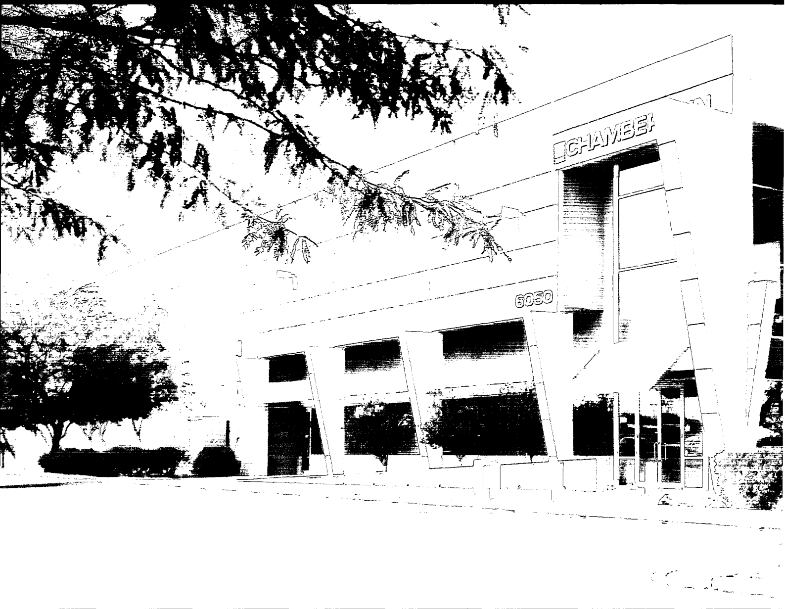
Chamberlain Distribution Center, Tucson, Arizona
