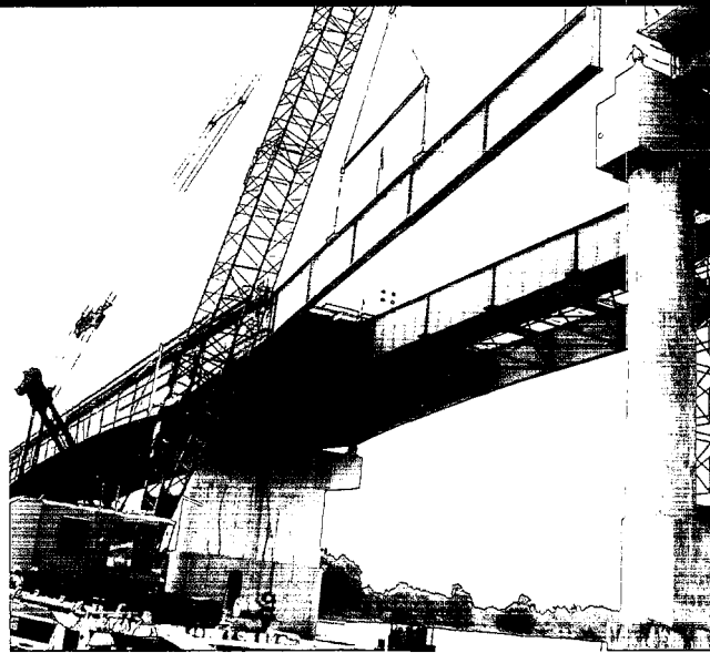
Trinity quickly fabricated 210 tons of bridge steel, allowing this damaged bridge in Oklahoma to reopen ahead of schedule.
