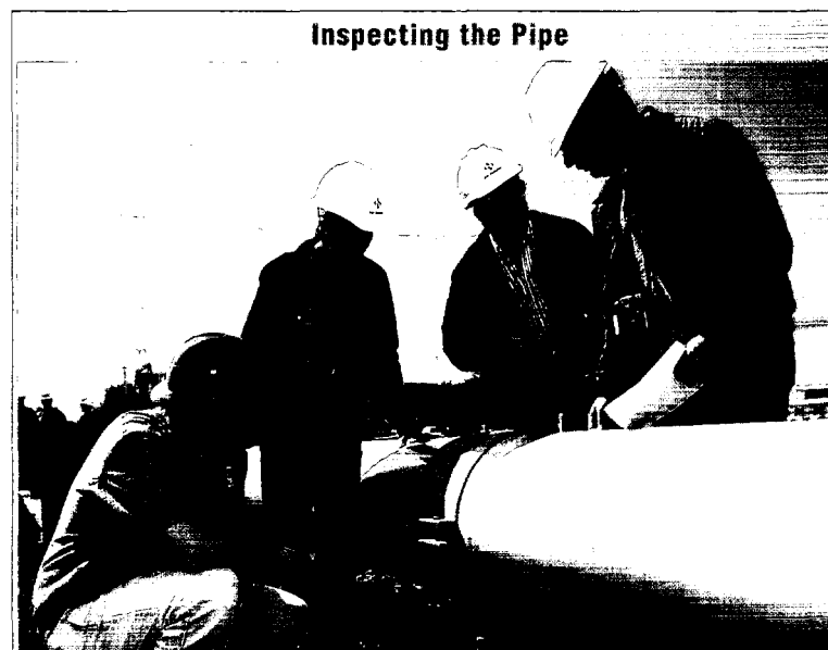
Federal and state regulators work with NW Natural to inspect pipelines for safety. Above (left to right) are Al Jones, pipeline safety engineer with the Washington Utilities and Transportation Commission; NW Natural Design Engineer Jodi Wright and Chief Engineer Bruce Paskett; and Steve Rieger, engineer with the U.S. Department of Transportation, Office of Pipeline Safety.
