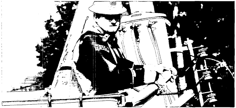
Above David Napolitano, line constructor, working on overhead wires in Staten Island. Left Daniel Huie, mechanic B, in an overhead training class at Con Edison's Learning Center.
