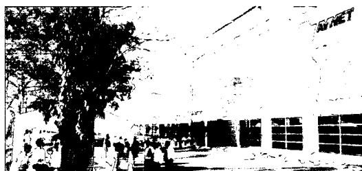
Electronics Marketing celebrates the grand opening of its 35,000 square foot sales, materials management and warehouse facility in Guadalajara, Mexico.
