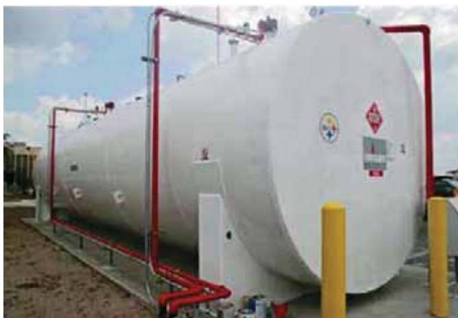
Figure 18.1: Aboveground Storage Tanks (ASTs) (Example)
