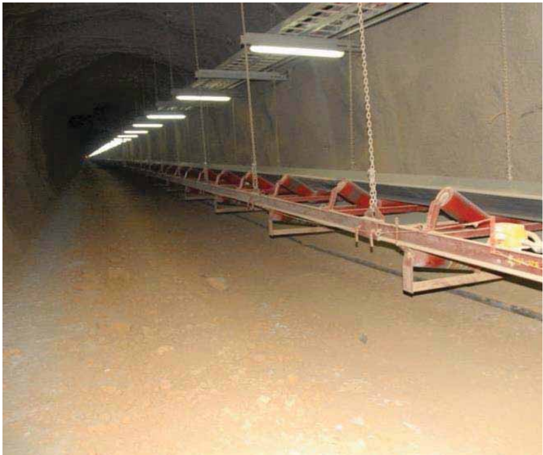
Figure 16.5: Typical Underground Suspended Conveyor Structure
