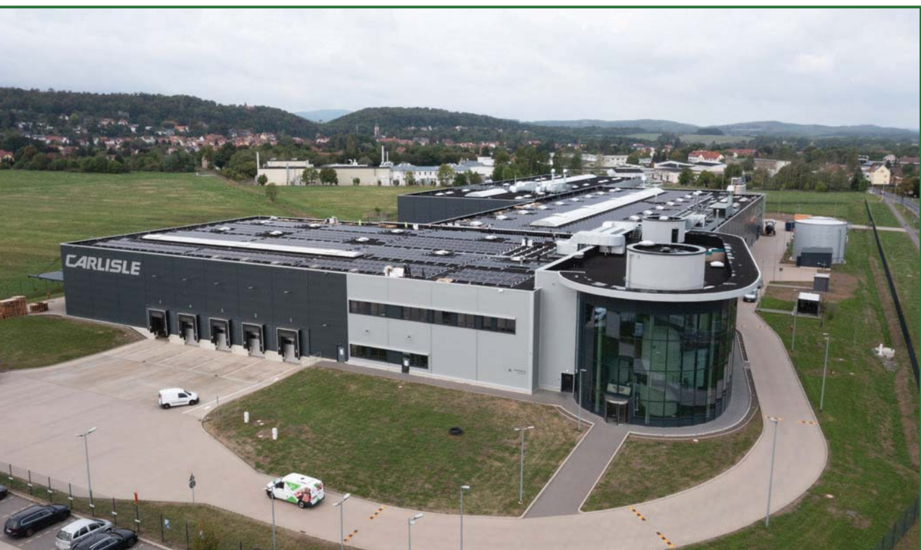
Carlisle's new plant in Waltershausen features rooftop solar panels that will reduce GHGs by almost 250 metric tons a year
