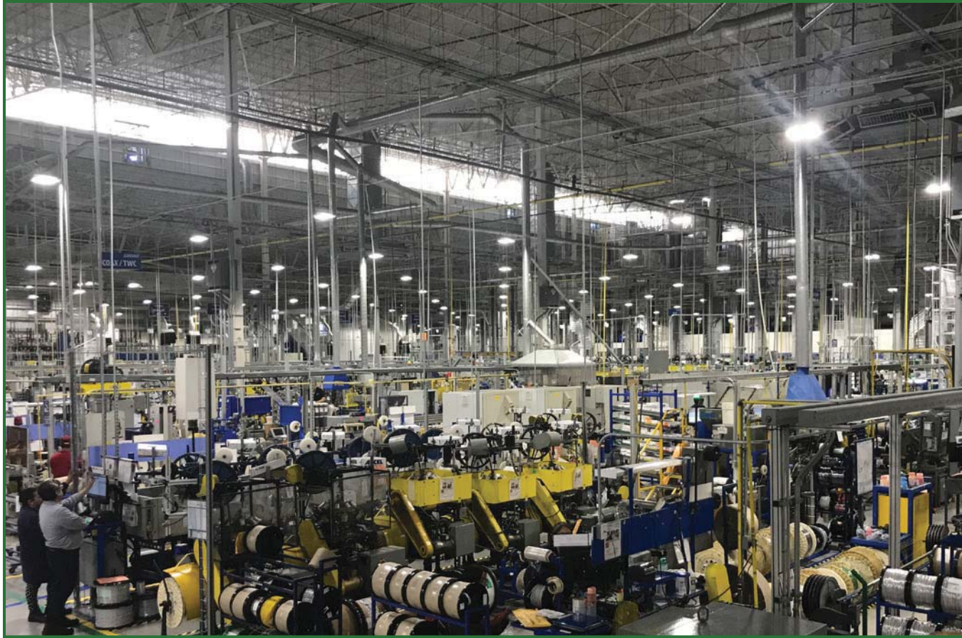
Recently installed LED lighting in our Nogales, Mexico CIT facility
