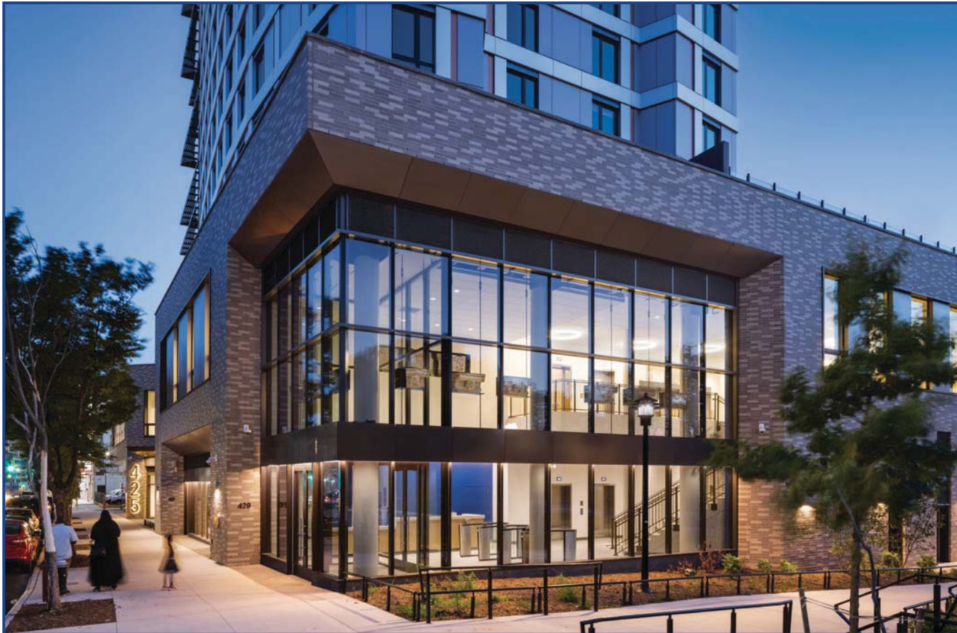
CWT's air barrier systems were installed at 425 Grand Concourse in Bronx, NY, the largest Passive House in the U.S. Credit © Albert Vecerka/Esto
