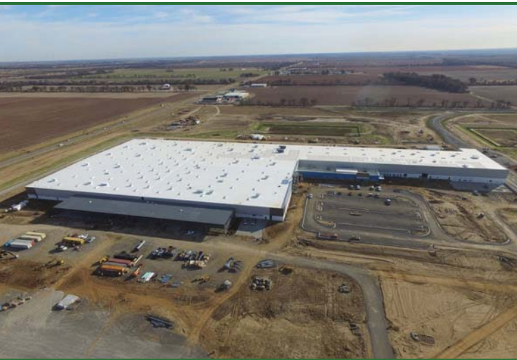
Construction of our new polyiso manufacturing facility in Sikeston, MO
