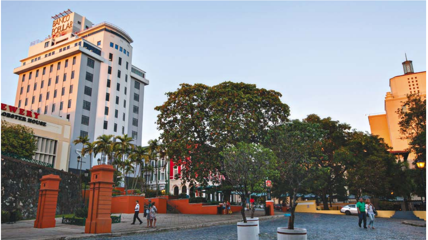
The inauguration of the former art-deco headquarters of Banco Popular de Puerto Rico on April 11, 1939 sent a strong message of local resilience near the end of The Great Depression, from which Puerto Rico recovered to transform its economy from agrarian to industrial. Today, the building in the historic Old San Juan hosts the Banco Popular Foundation, a full-fledged branch and an exhibition hall where it explores socioeconomic issues of Puerto Rico.
