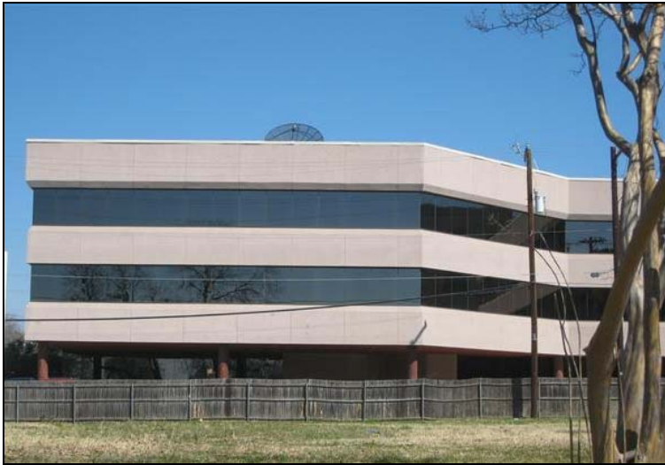
GSA Office 4211 Cedar Springs Drive Dallas, Texas
