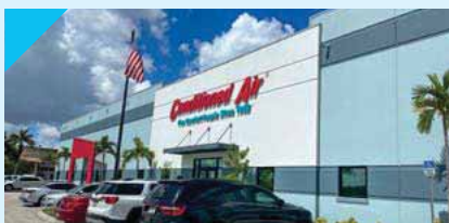
CONDITIONED AIR Fort Myers, FL
