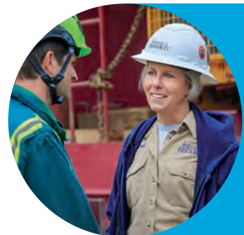
Seneca employee speaks with a contractor about a Well Done Foundation (WDF) plugging project in Bradford, PA. Seneca provided funding to WDF, a nonprofit aimed at plugging orphaned and abandoned wells, to support WDF's first orphaned well plugging in PA.
