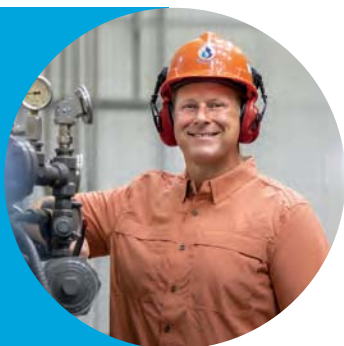
Supply employee inspects an upgraded compressor unit in Mercer County, PA. New unit equipment helps to improve efficiency and lower emissions.
