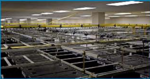
Data Centers Fiber Optic Replacement
