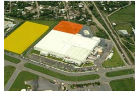
New Linares Pump Plant
