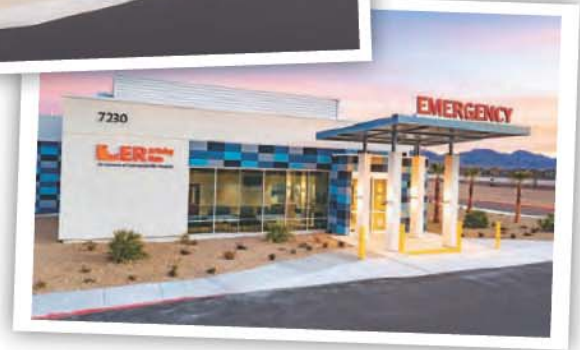
ER at Valley Vista, an extension of Centennial Hills Hospital Medical Center
