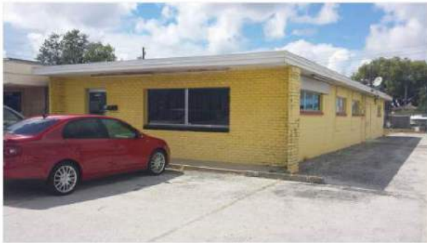
Ugly on the outside - functional on the inside
