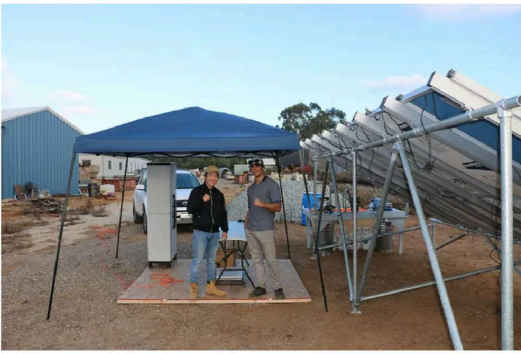
Our team working on our first installation.
