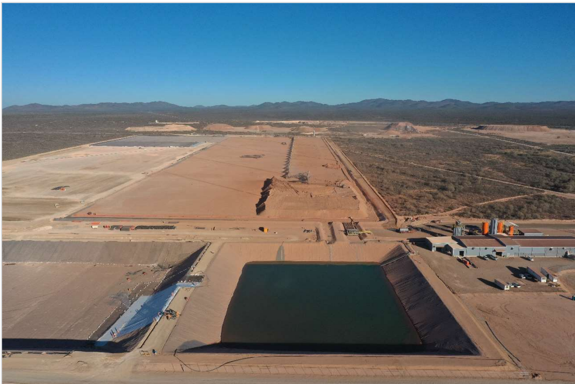
Figure 2: Pregnant Solution Pond (front), Heap Leach Pad (back), Merrill-Crowe Plant (right)
