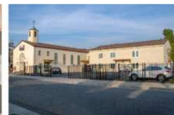
Completed Project: Genesis Worship Center
