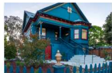
Completed Project: 501 River
