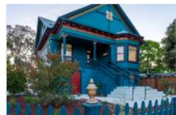
Completed Project: 501 River
