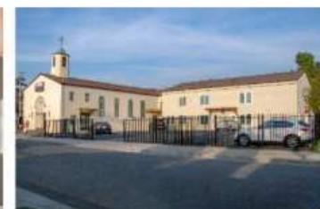
Completed Project: Genesis Worship Center
