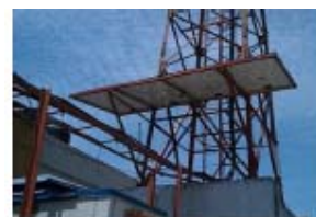
Rooftop Solar Panels
