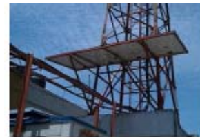
Rooftop Solar Panels
