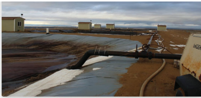
Traditional industrial water evaporation pit, used to separate sludge from water.
