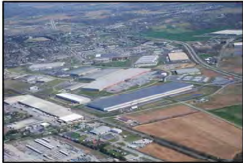
Commercial development in the northern study area, adjacent to the Borough of Chambersburg
