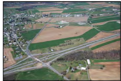
View of the Marion Interchange and the southern part of the study area illustrating mainly agricultural land use
