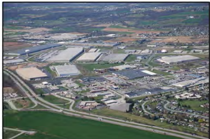
Development around the I-81 Wayne Avenue Interchange
