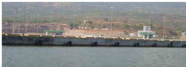
Puerto La Union Wharf from SE
