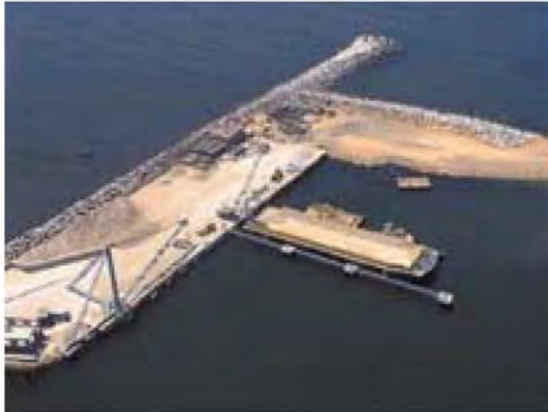
Ensenada Petroleum Terminal
