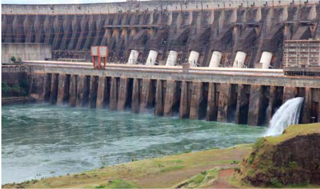
The Itaipu Dam on the border of Brazil and Paraguay provides electricity for both countries. Brazil may have to tap its large hydroelectric potential to meet its increasing energy needs.
