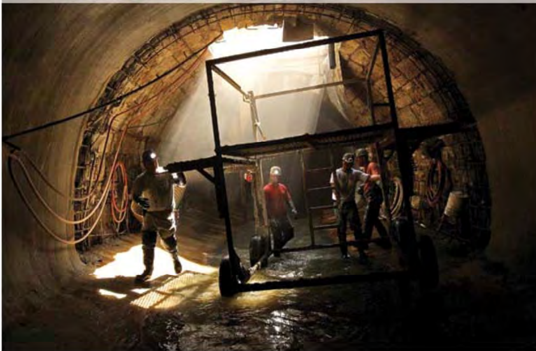
Workers restore a section of storm sewer about 25 feet below ground in St. Louis, Missouri.
