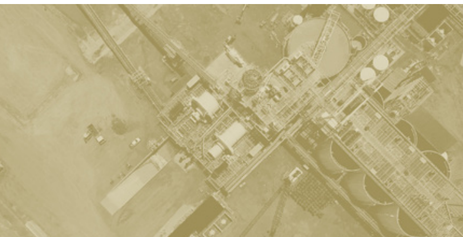
Houndé Gold Mine Overhead view of processing facility
