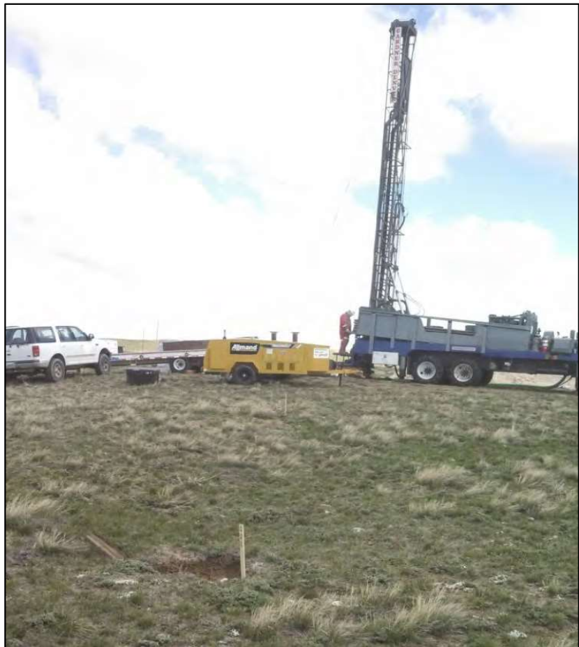
Figure 13. Photo of URE Confirmation Drilling
