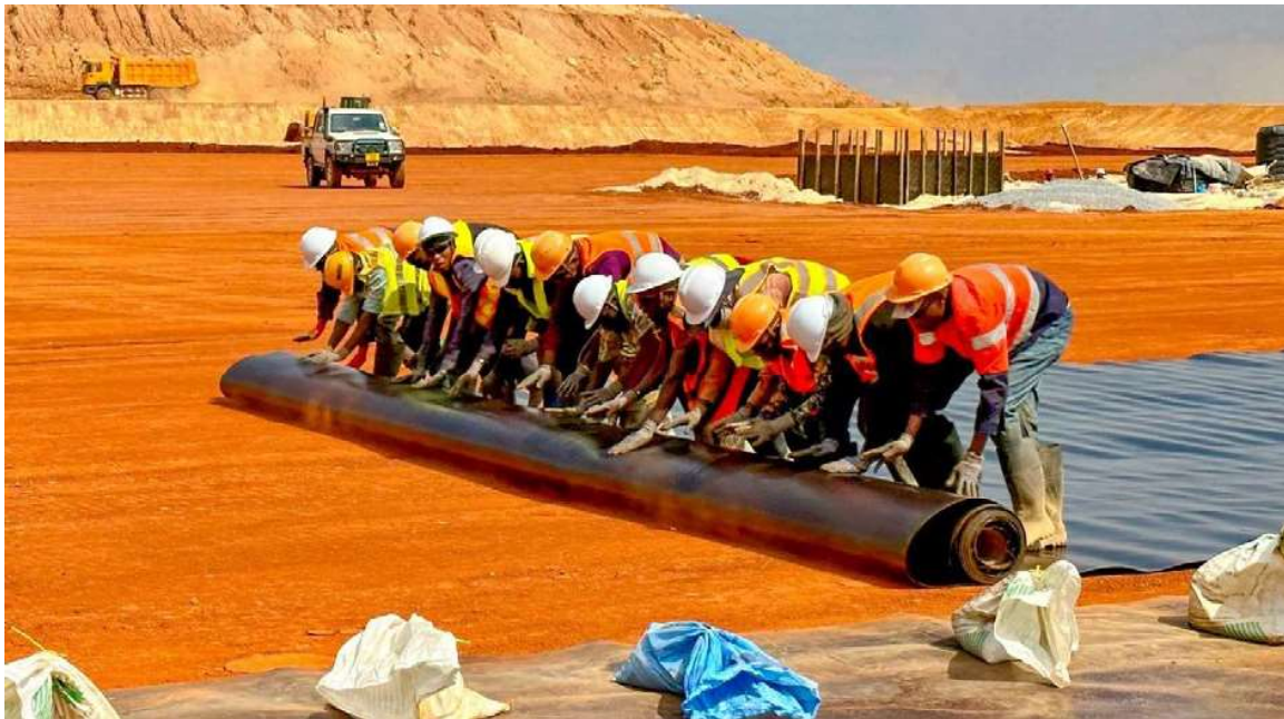
Figure 5b: Buckreef Gold Tailings Storage Facility Expansion liner installation at TSF 2.2 (Q3 2023)
