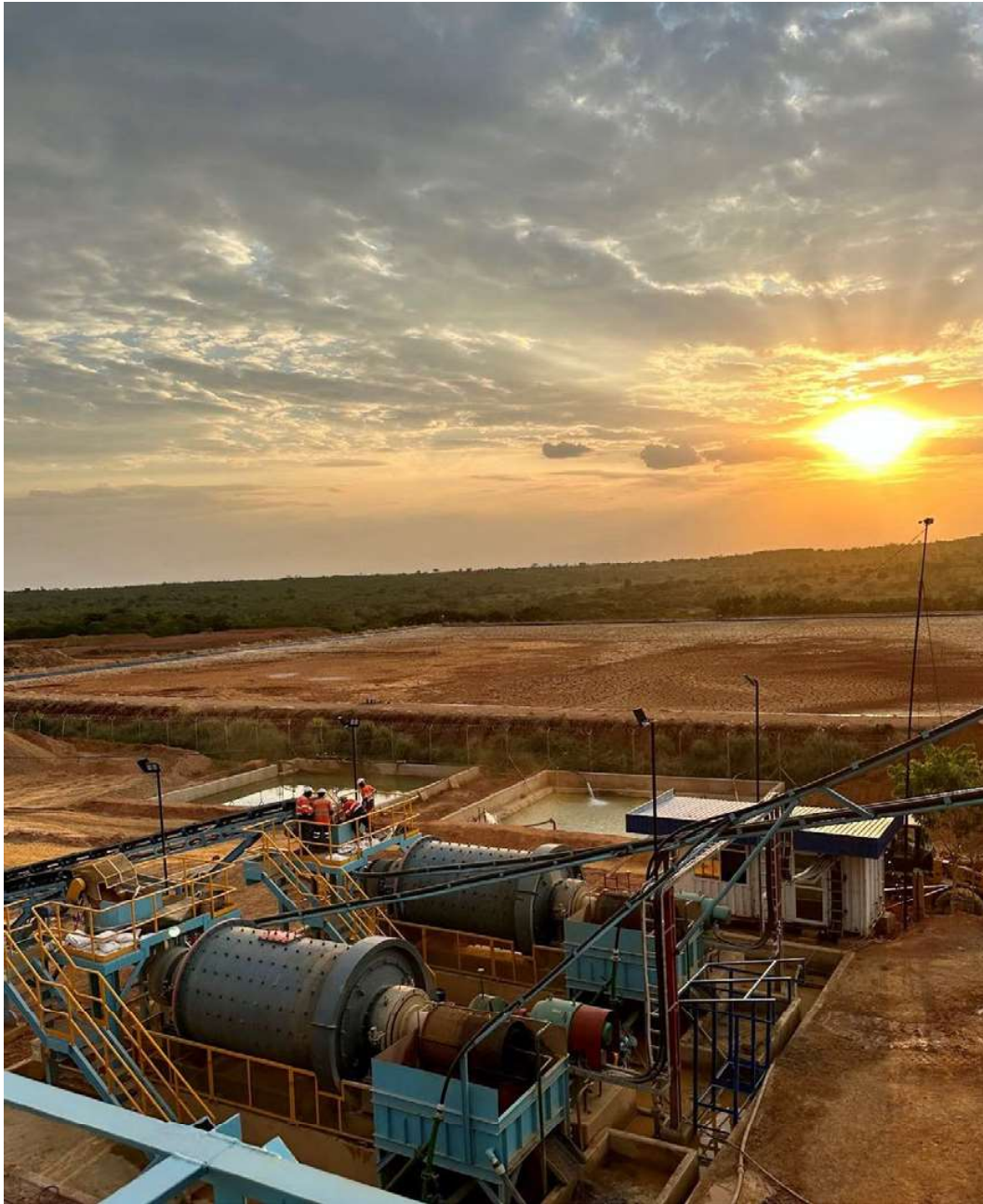
Figure 4: Buckeef Gold Expanded 1,000+ tpd Processing Plant, showing installation of two new 360 tpd ball mills (Q1 2023)
