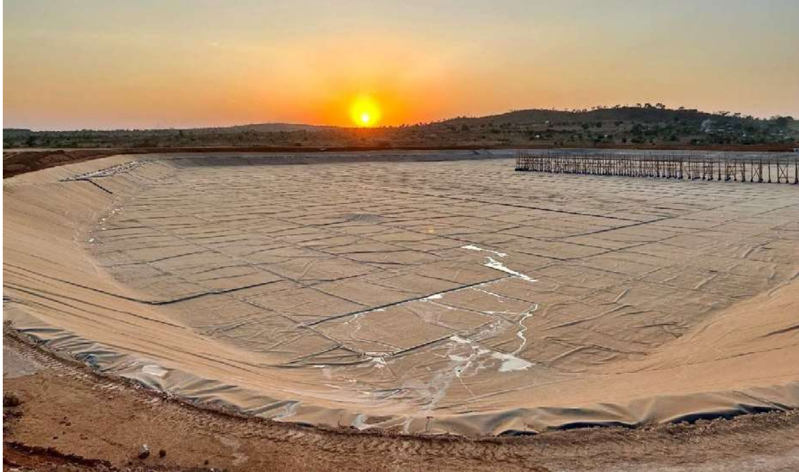
Figure 5b: Buckreef Gold Tailings Storage Facility Expansion liner installation at TSF 2.2 (Q3 2023)
