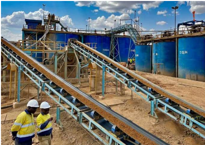
Figure 3: 1,000+ tpd Processing Plant at Buckreef Gold Mine, showing new CIL tanks and conveyor feed to the new ball mills (Q3 2023)
