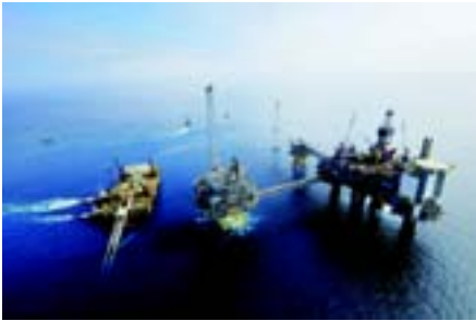
Langeled passes Sleipner. Sleipner is a hub in the Norwegian gas machine. The latest addition is Langeled and the picture was taken during the pipelaying process
