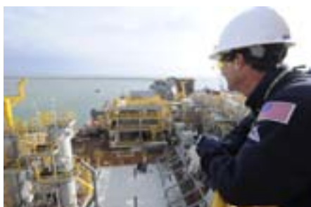
US Gulf of Mexico. At the yard in Corpus Christie, work is underway to complete the Tahiti platform.
