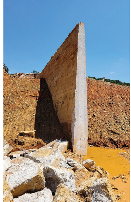
1912 concrete core wall
