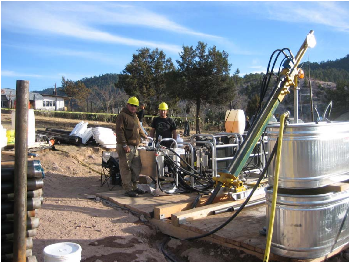
Photo 13.1 Hydracore Gopher Drill at Drill Hole LBDDH-001
