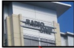
Radio One Headquarters Silver Spring, Maryland
